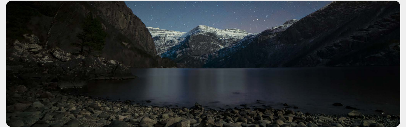
The Bremanger dam in Vestland county, western Norway, was targeted by a cyberattack, which resulted in the sluice gates being left wide open for several hours. Photo: Shutterstock
